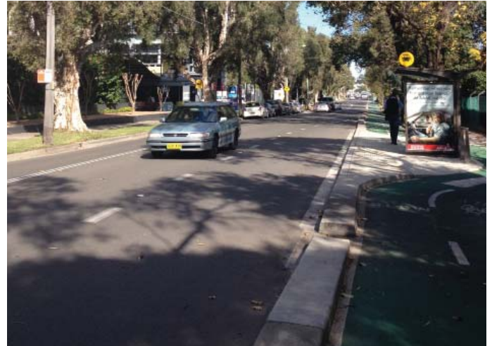
Bourke Road Separated Cycleway
