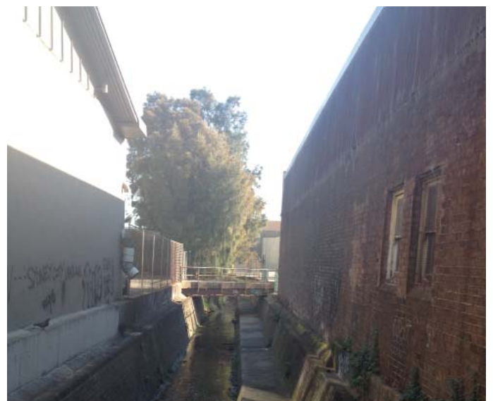
Open Culvert Condition in Northern Study Area
