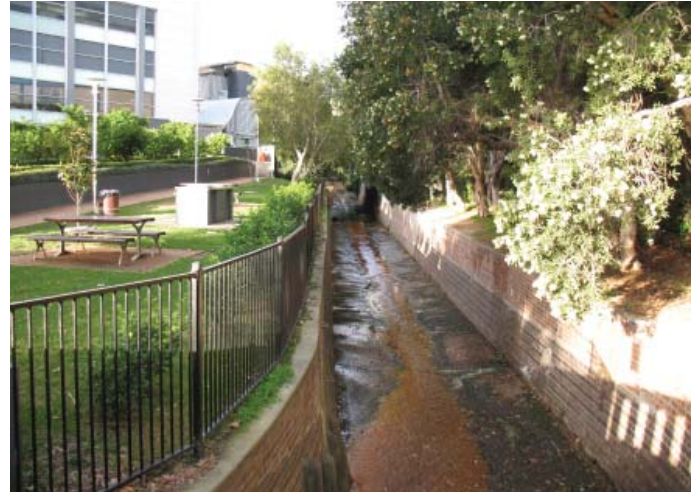
Open Culvert Condition
