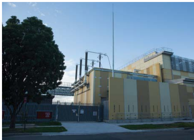
Beaconsfield West Substation on Burrows Road
