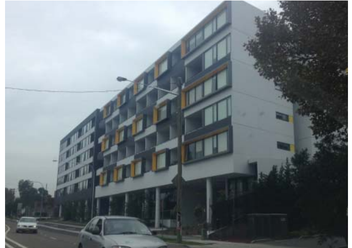
Apartments on Gardeners Road, Mascot
