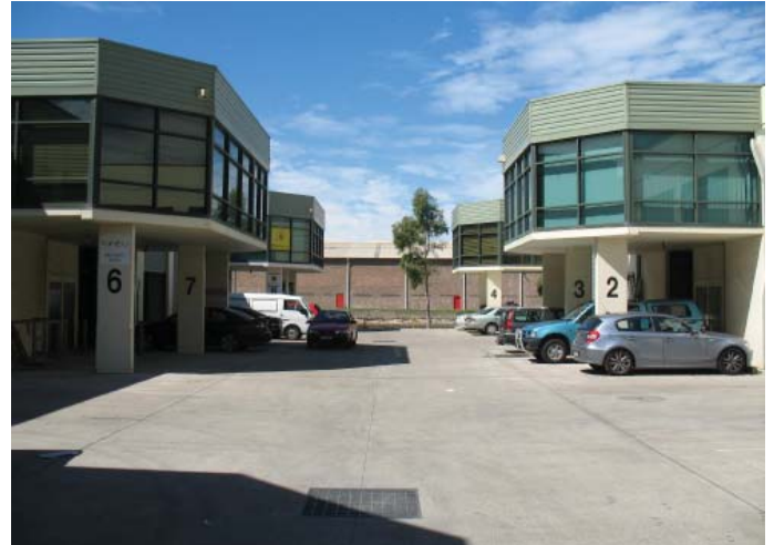
Strata Industrial Units
